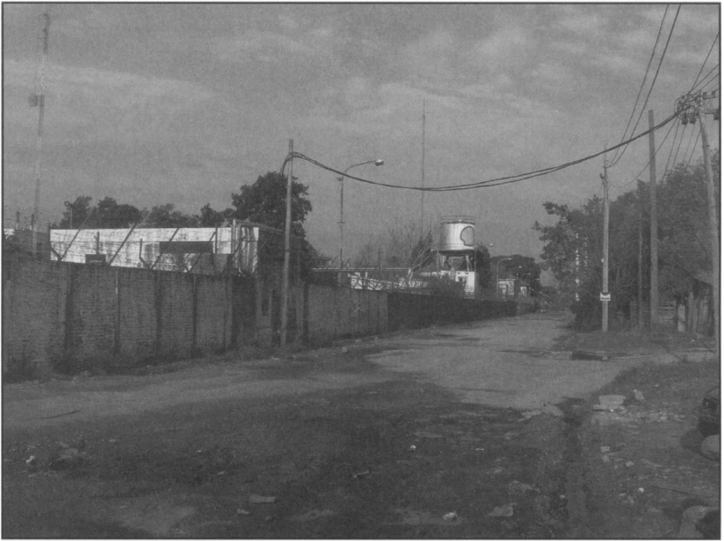
Photograph 2. The walled petrochemical compound as seen from Flammable, June, 2004.
