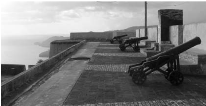
Cannons at Fort Charlotte, pointing inland
