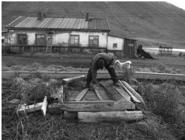
Figure 2. "Meat pit" permafrost cellar. Enmelen, Chukotka. Photo by Sveta Yamin-Pasternak. A color version of this figure is available online.
